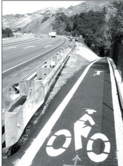
New Bike Detour Northbound on the Cuesta Grade (opened February 2004).
