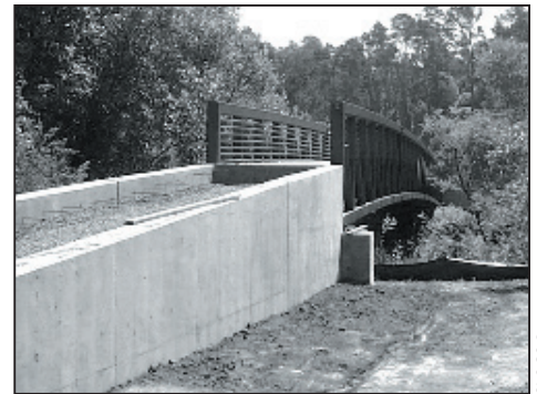
The new Santa Rosa Creek Bridge in Cambria
