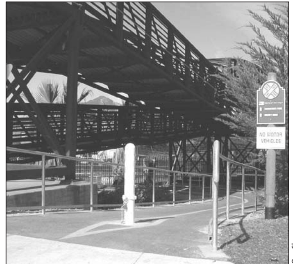
Jennifer Street bridge entrance to the Railroad Safety Trail.
